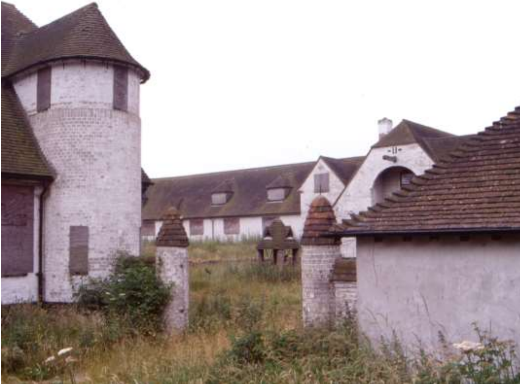
Existing Building looking South, before the redevelopment
